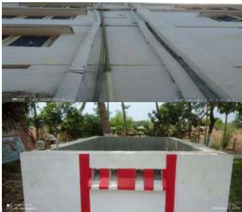
Fig 3: Rainwater Harvesting Recharge Tank
